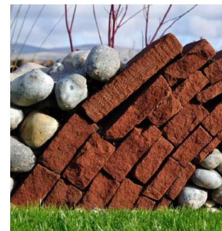
Combinations of local stone – red sandstone and river pebbles – create complementary features
